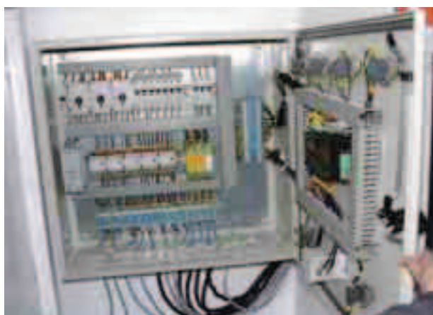
Fig. 3. A control cabinet with electrical protection elements and a PLC-HMI controller installed on the cabinet door
