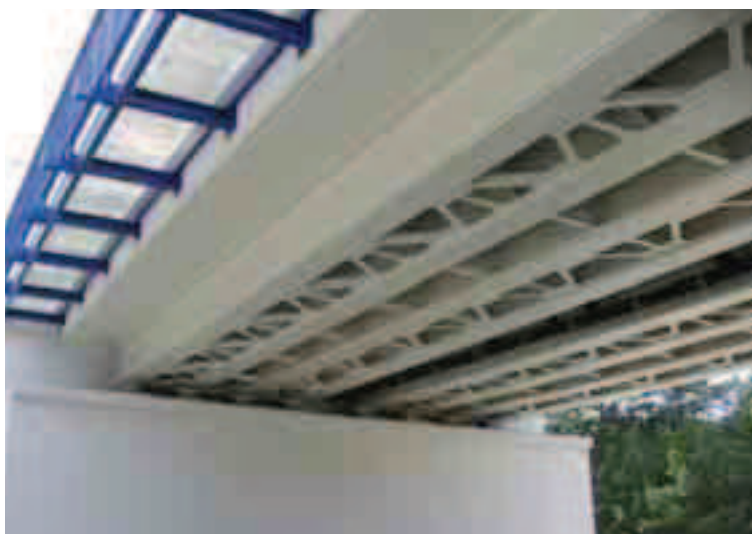
Fig. 1. The modernized viaduct No. KNI 140 070 composed of two separate spans, located at the PCM Line, Poland. Bottom view on the main beams and bracing
