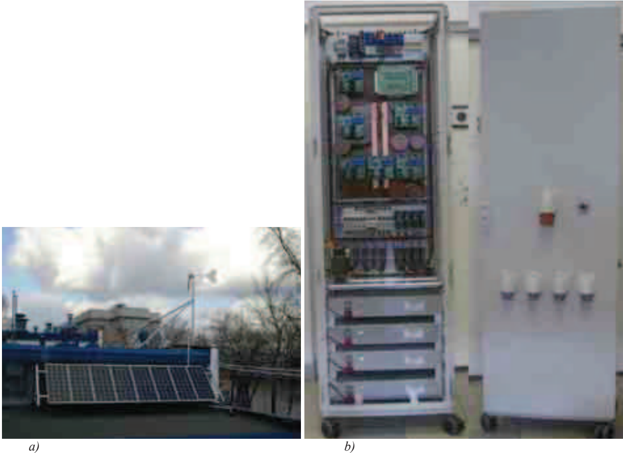
Fig. 2. View of photovoltaic panels (a) and control cubicle (b) of the charging station demonstrator
