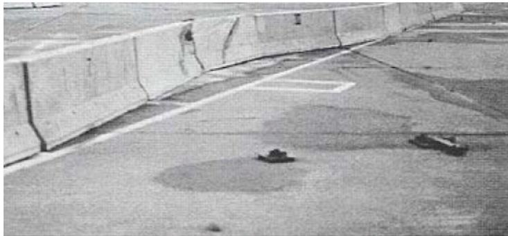
Fig. 2. Concrete barrier displacement on impact of a vehicle [2]
