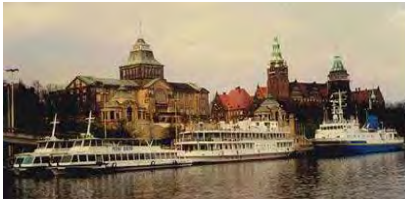
Fig. 1. The view on Waly Chrobrego Quay alongside Odra River
