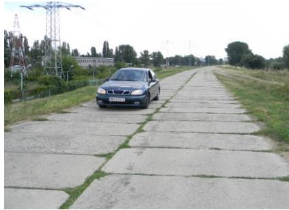
Fig. 5. Test road section with “rough” surface
