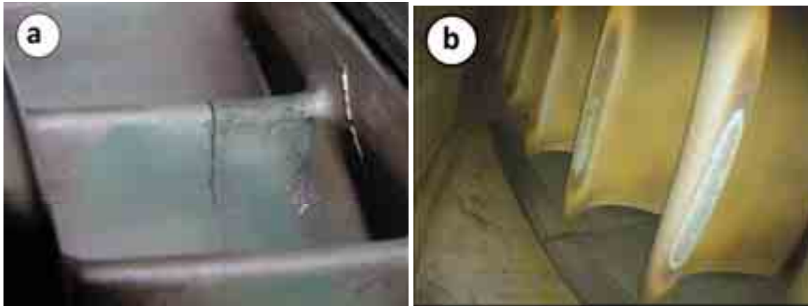
Fig. 1. Forms of thermal deterioration of gas turbine blades: a) overheating of the blade material visible as discoloration of surface colour to pale blue and glaucous, b) local melting of the protective coating
