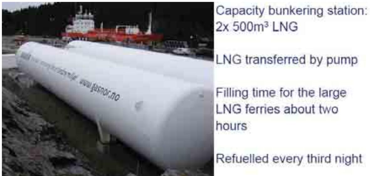
Fig. 5. LNG bunkering station at ferry berth for m/v Bergensfjord [10]
