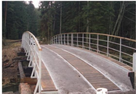
Fig. 1. Adaptation of a 20-metre long BLG-67 support bridge span to non-military traffic in Kletno, gmina Stronie Śląskie, Kleśnica creek: a) deployment of BLG-67 b) span adaptation
